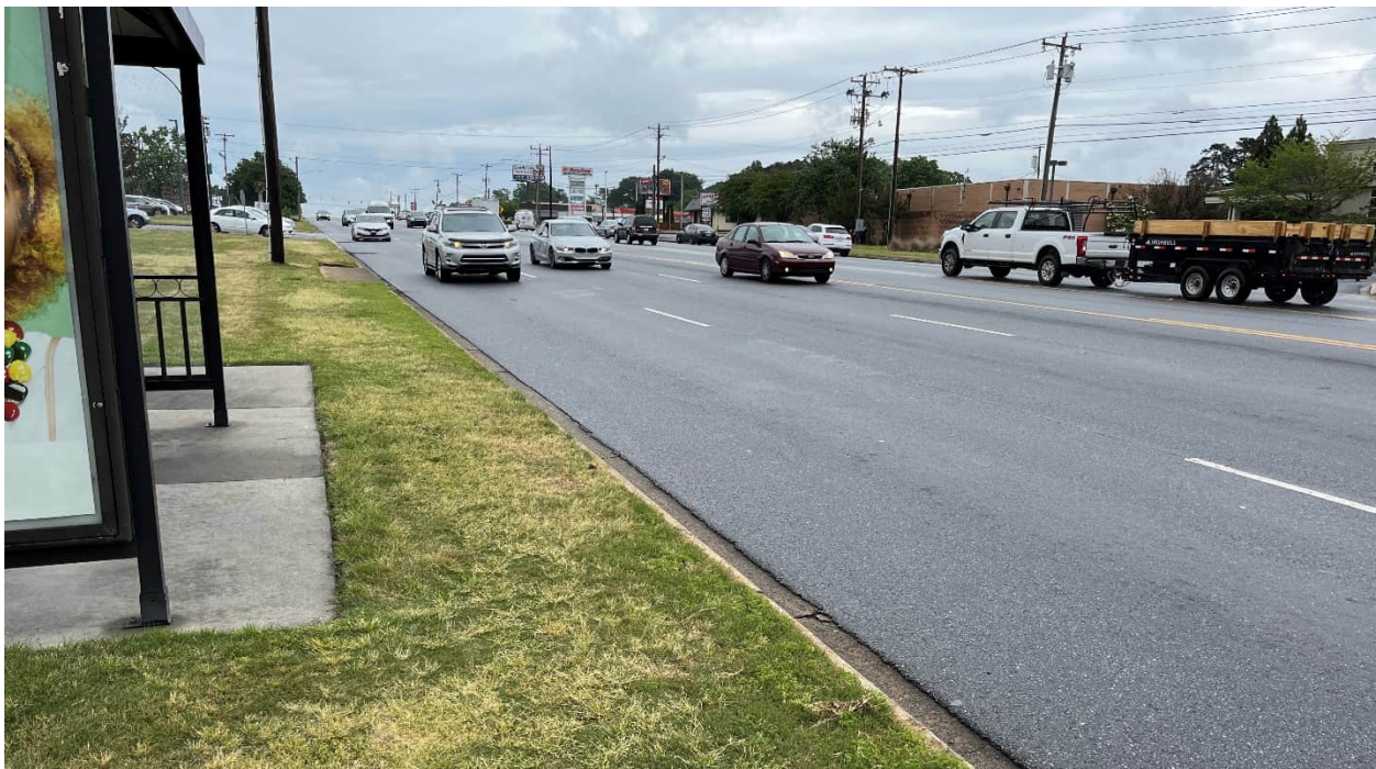
Looking northbound along US 29 near Hampton Village Shopping Center. Multiple driveways along this segment with no significant access management measures in place.
