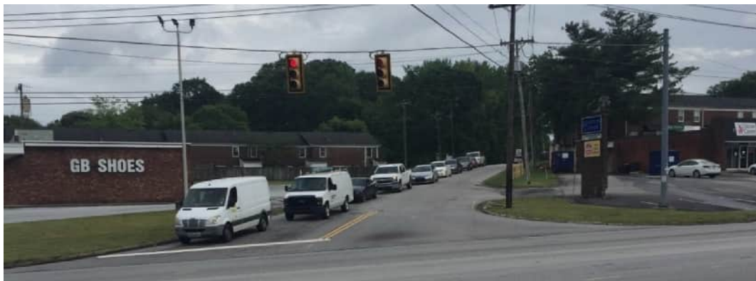
Looking at the westbound approach of Watson Road. Queues observed on side street. No pedestrian accommodations present are present at intersection.
