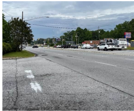
Looking northbound along US 29 toward Tappan Dr
