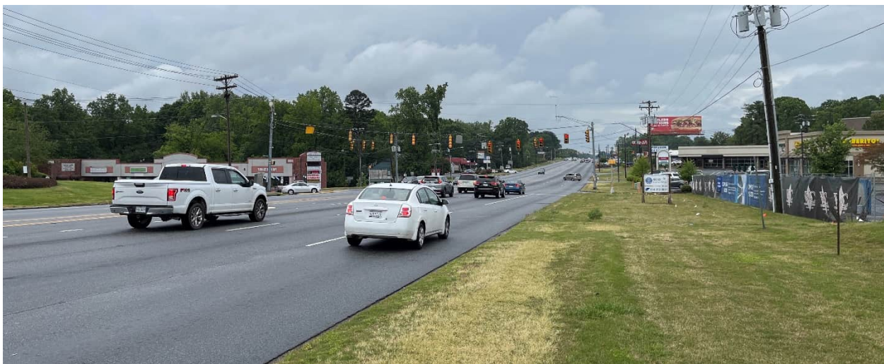
Looking southbound along US 29 towards East Lee Road. Vehicles approach intersection heading downhill and would likely benefit from a nearside signal head.
